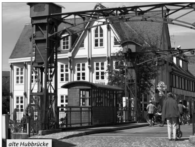
alte Hubbrücke in Plau am See
